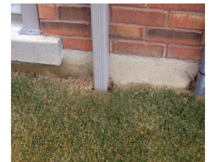
These downspouts are connected to the underground municipal sewer system.
