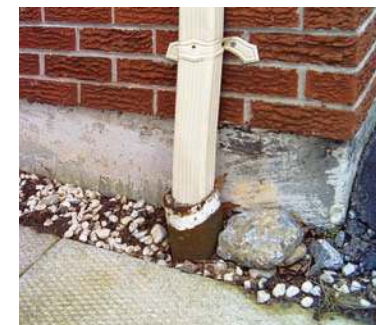
These downspouts are connected to the underground municipal sewer system.
